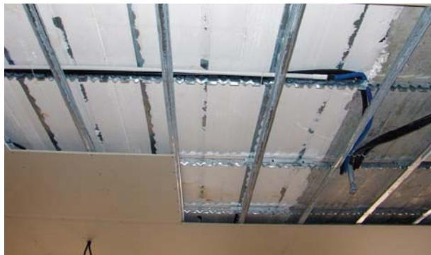
**Model C** - for internal dry finishing with built-in metallic profiles exposed with interaxis 30 cm - panels are not fitted with any metal grid as they are meant to be left raw or covered with gips boards, false ceilings or any kind of internal dry finishing.
