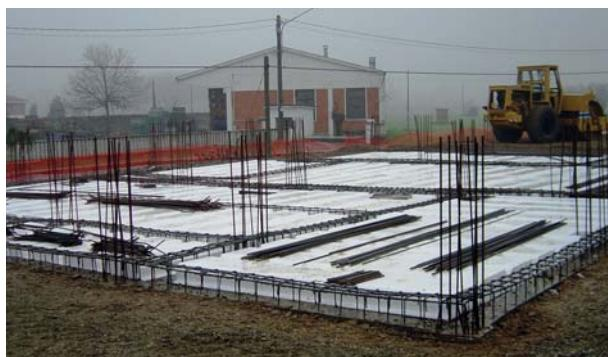
**Model S** - for ground floor insulated crawl space - panels are manufactured of EPS only and thus they are not self-supporting; they are layed as crawl space on the ground floor to grant natural ventilation and insulation without thermal bridges. Layed on a sand-bed or as overlaid floor to pre-existing structures to be replaced.
